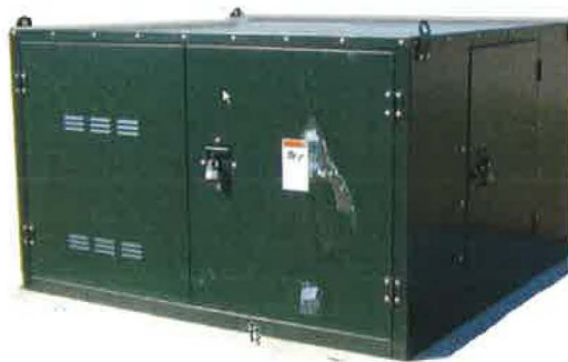
Figure 3-3, Typical Padmounted Deadfront Sectionalizing Switchgear
