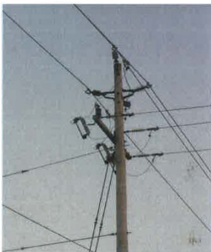
Figure 3-1, Typical Fused Tap Framing
