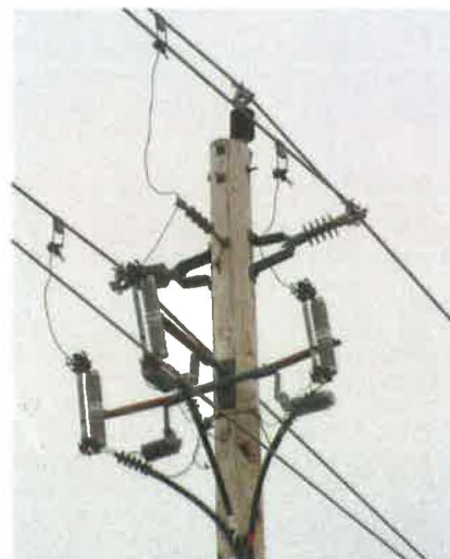
Figure 3-2, Typical Fused Riser Framing
