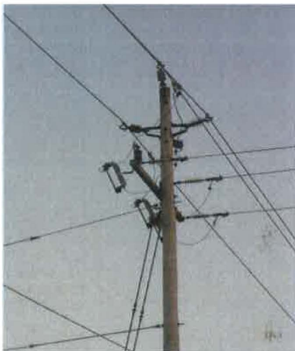
Figure 3-1, Typical Fused Tap Framing
