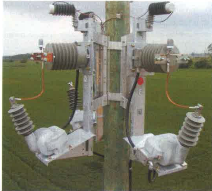
Figure 6-1, Typical Primary Metering Unit
