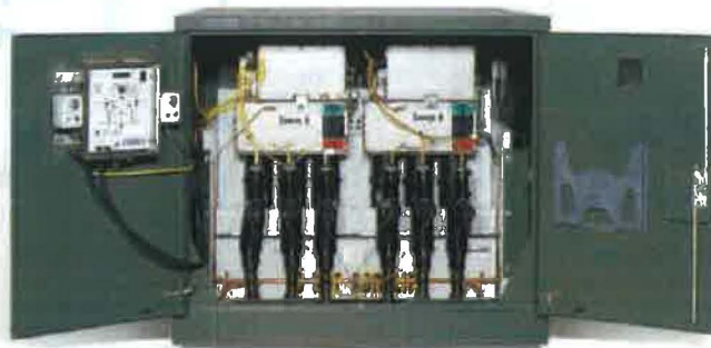
Figure 3-5, View of Switchgear Interrupter Switch Compartments
