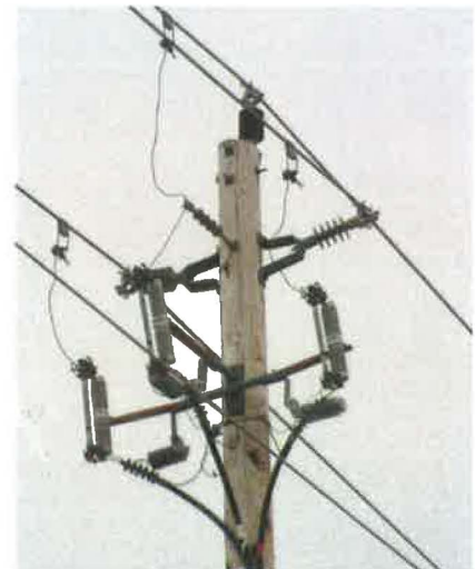
Figure 3-2, Typical Fused Riser Framing
