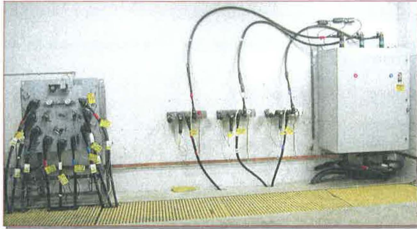
Figure 3-6, Indoor Switching Vault
